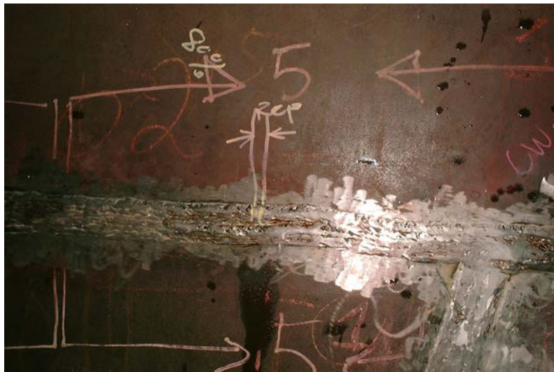
Fig. 4 shows a welded area completed & DP examined
