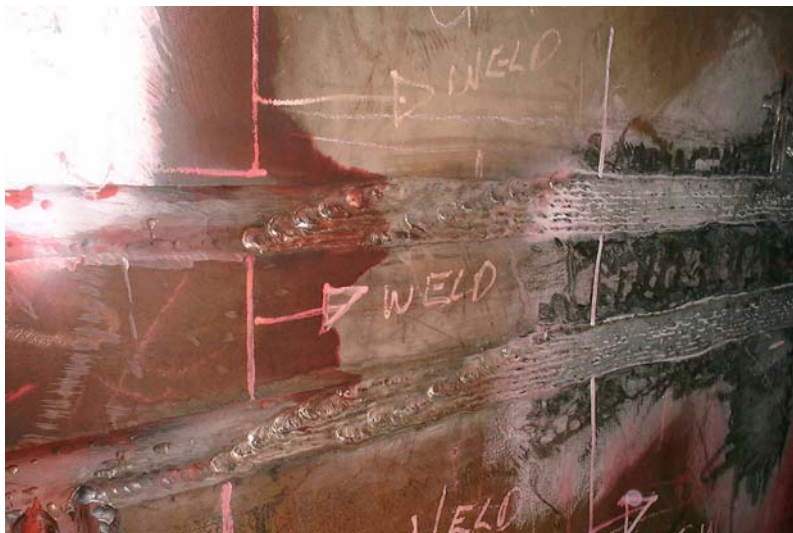
Fig. 2 shows the combined excavation for the equator areas during welding
