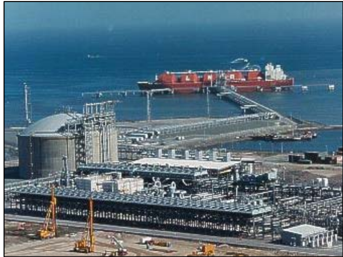
Figure 1: LNG facility showing storage tank, pier and ship
